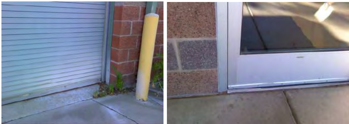
Figure 50: Gaps in Building Envelope at Transit Administration
