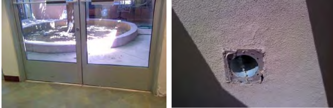
Figure 13: Gaps and openings in building envelope at the Fort Marcy Recreation Complex
