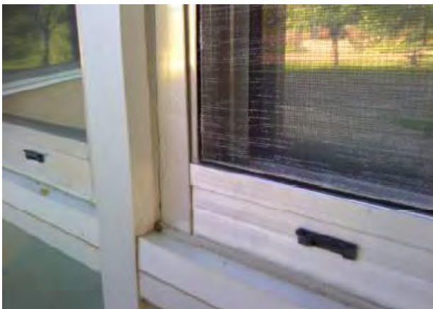
Figure 47: Additional Gaps in Building Envelope at Siringo Complex Warehouse
