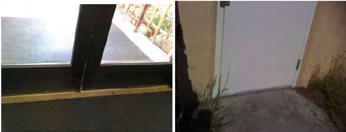
Figure 56: Gaps in Building Envelope at the Water Division Office
