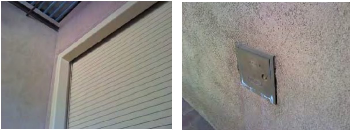
Figure 35: Building Envelope Gaps at SFCC
