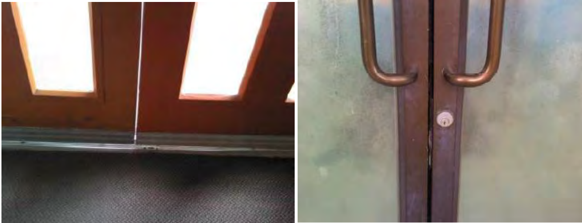
Figure 7: Gaps in building envelope at Alto Complex
