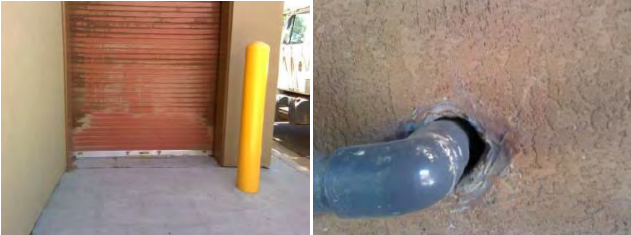
Figure 54: Gaps in Building Envelope at Canyon Road Water Treatment Plant
